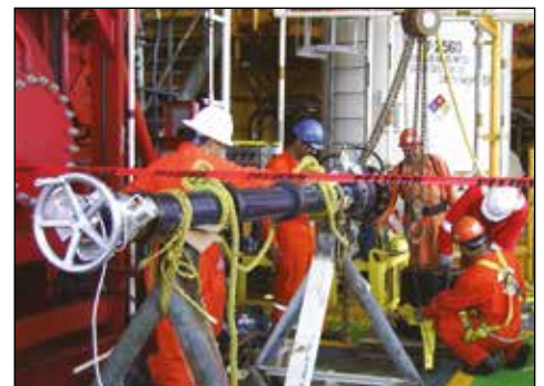
▼ CHT2000 hot tapping offshore application.
