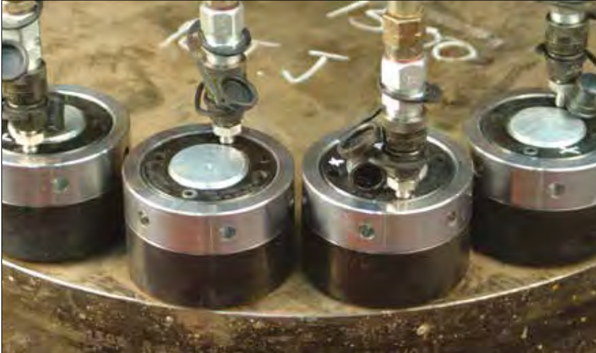
▲ Tensioning with hydraulic nuts.
