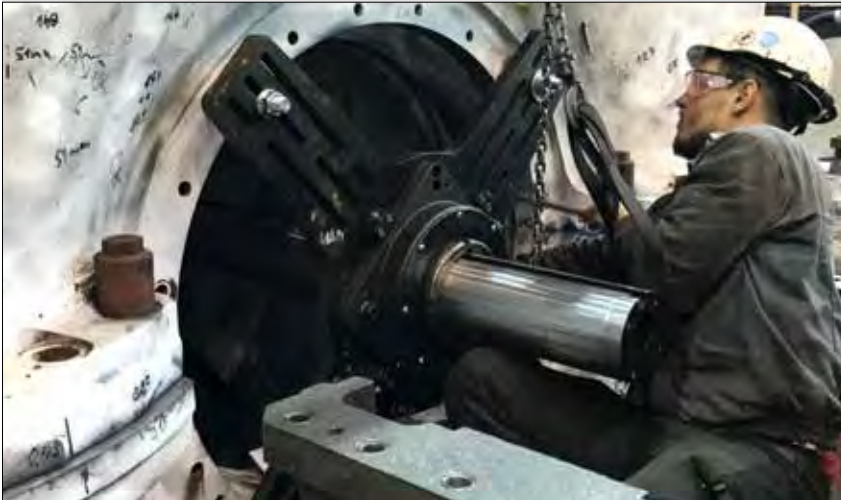
▲ Pipe cutters and weld preparation.
